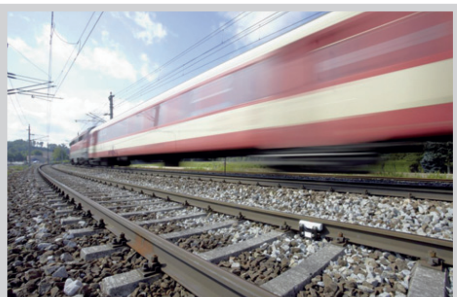
Figure 2: Axle counting technology on modern main lines
